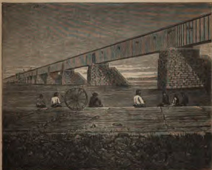
Fig. 249.—[The Victoria Bridge, from a Photograph.]
